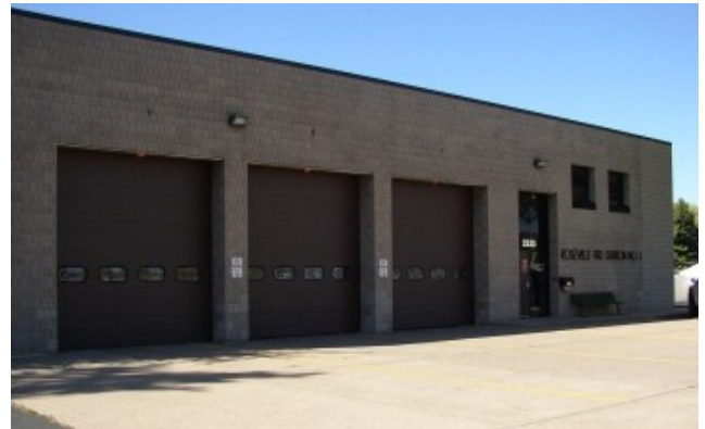
Roseville Fire Station 1 has a serious mold problem
