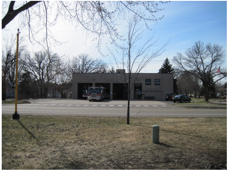
Fire Station 3 and other Roseville Fire Stations do not have sprinkler systems.
